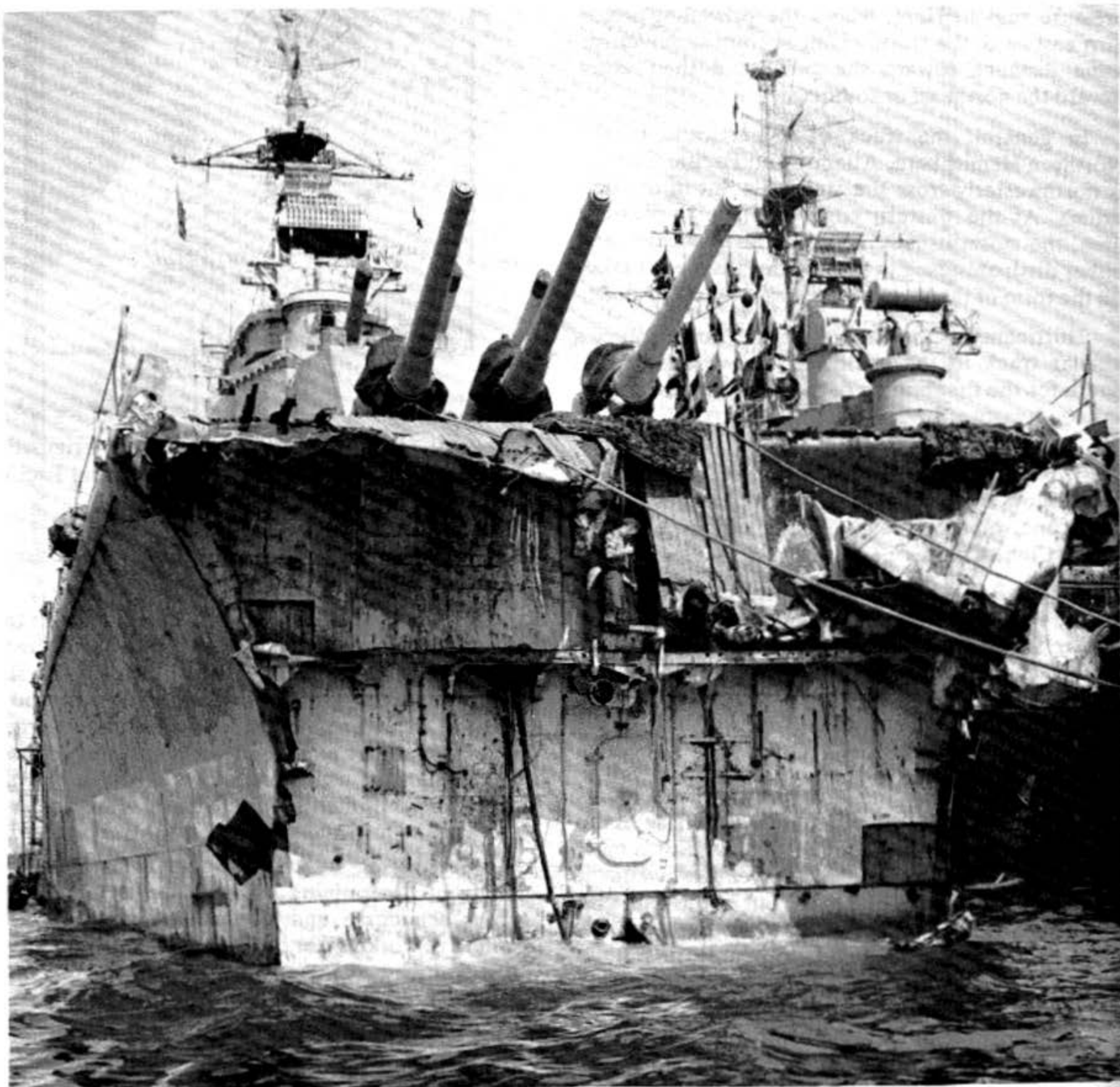
Figure 9-5. Bow of USS Pittsburgh ripped off in a typhoon. 112.66
